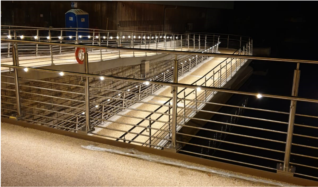
Chobham Bridge, Surrey
